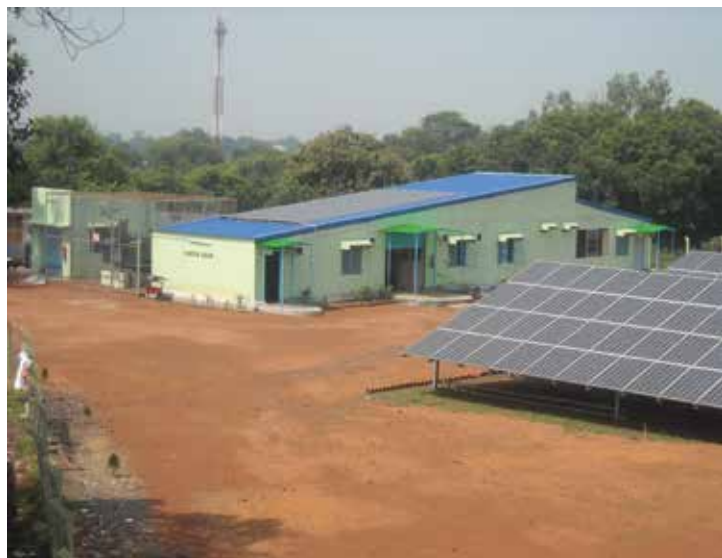
Solar plant at Seebpore receiving station.
